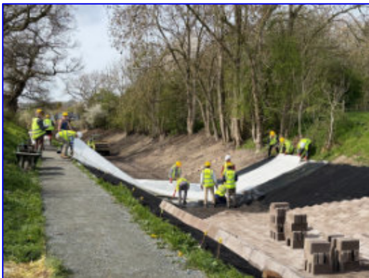
Lining and blocking in progress on the Phase 2 section of canal
