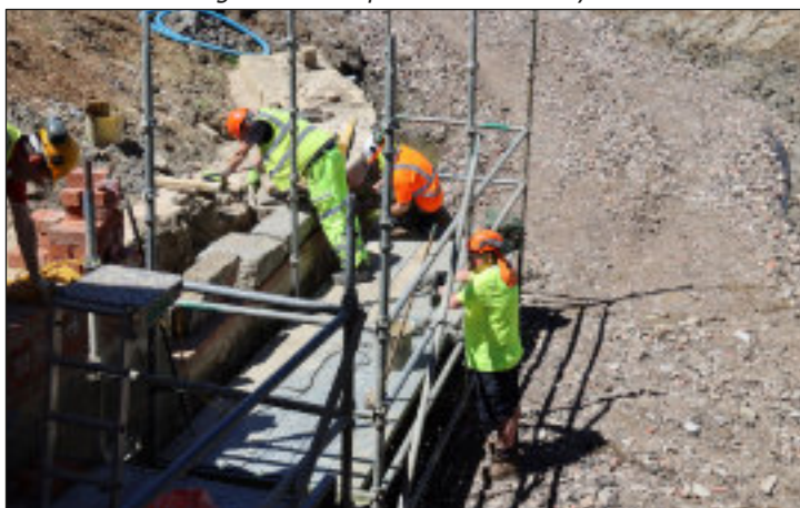
Rebuilding begins on the towpath side wing wall beyond the tail bridge
