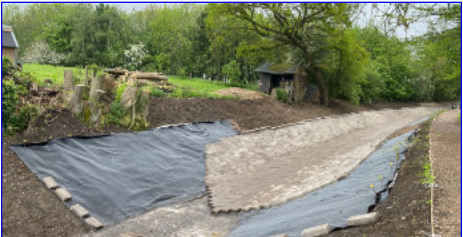
Pictures taken on the Thursday afternoon and Sunday afternoon show how much progress was made with lining and blocking during the May working party
