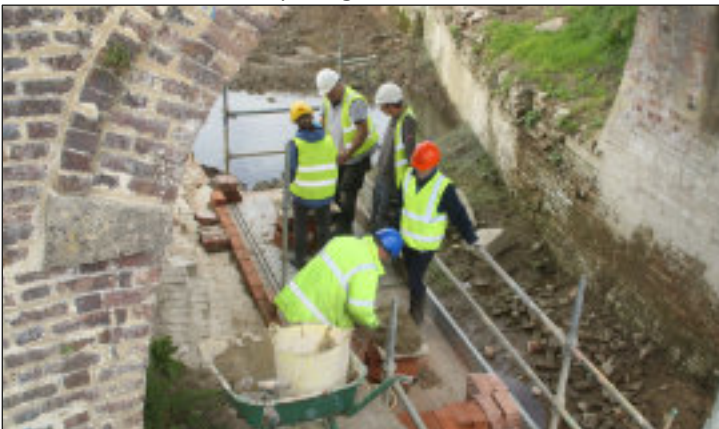
Bricklaying lessons on the towpath wall under the tail bridge
