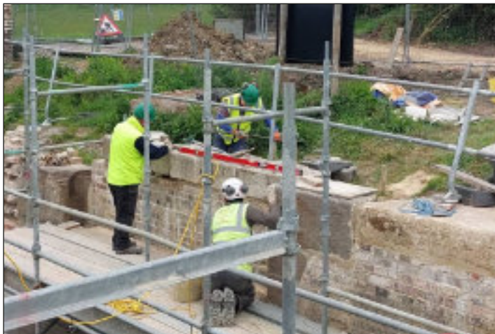
Laying coping stones at John Robinson Lock on the Cotswold Canals, and (below) the finished job
