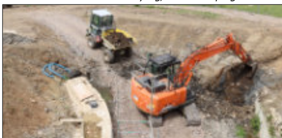
Demolishing the offside wing wall ready for rebuilding this summer
