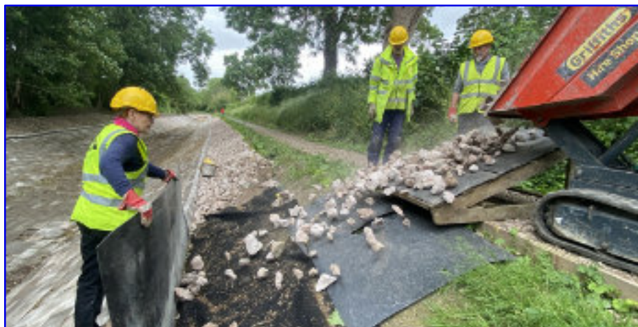
On the towpath side of the canal, the riprap stone can be delivered by tracked power barrow (above), but on the offside (below) it has to be done with buckets and wheelbarrows
