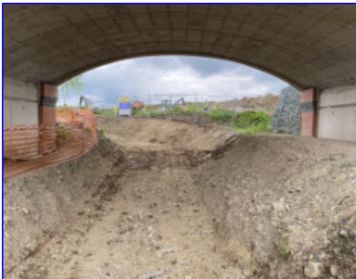
Schoolhouse Bridge with spoil to be cleared from underneath and each side of the bridge, and (below) with the channel completely cleared
