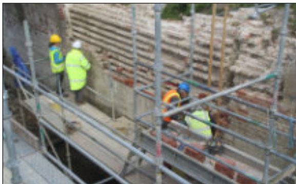
Rebuilding the offside wall between lock and tail bridge...
