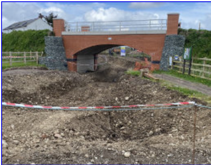
Schoolhouse Bridge with spoil to be cleared from underneath and each side of the bridge, and (below) with the channel completely cleared
