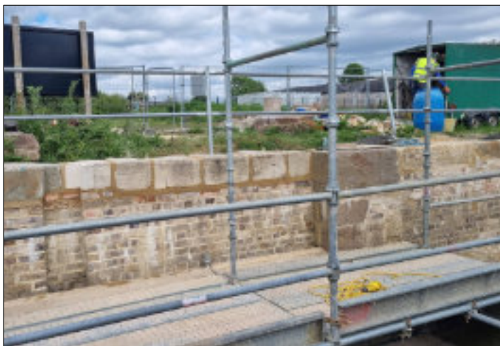
Laying coping stones at John Robinson Lock on the Cotswold Canals, and (below) the finished job
