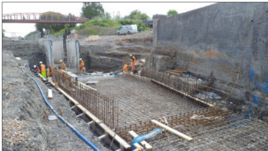
Constructing the new concrete channel walls at the old railway bridge site below the new Keith Ayling Lock
