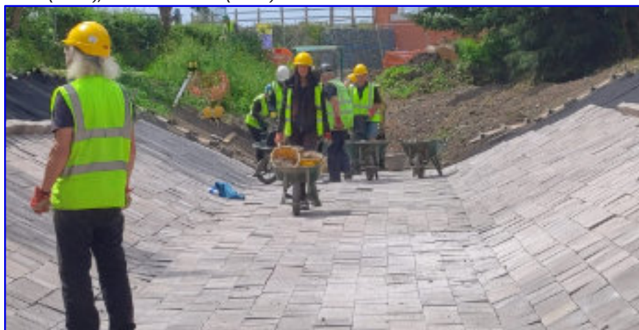
On the towpath side of the canal, the riprap stone can be delivered by tracked power barrow (above), but on the offside (below) it has to be done with buckets and wheelbarrows
