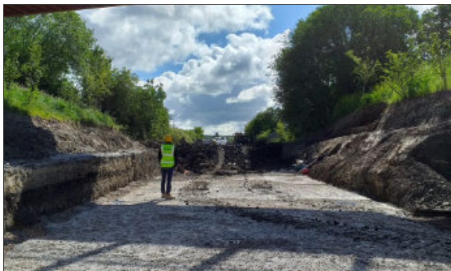
Next job: the concrete canal bed under the Trans Pennine Trail bridge. The initial blinding layer has been laid
