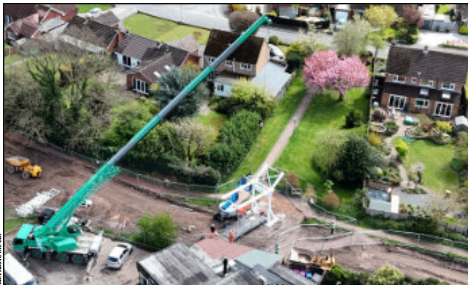
Some very clear practical restoration progress with the new liftbridge by Tamworth Road on the Lichfield
