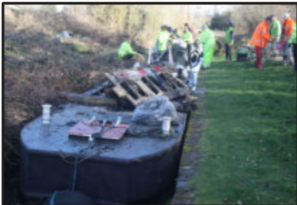
The junk pulled out is loaded onto work boats for disposal
