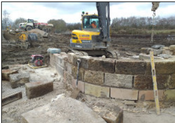
Building the stone walls of the narrows at the canal basin entrance
