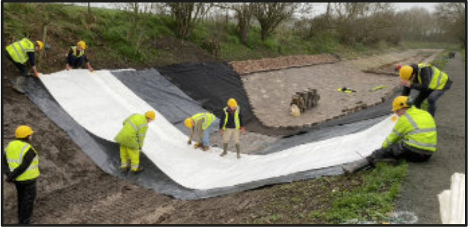
Laying the waterproof liners, with a section already covered with blocks visible beyond
