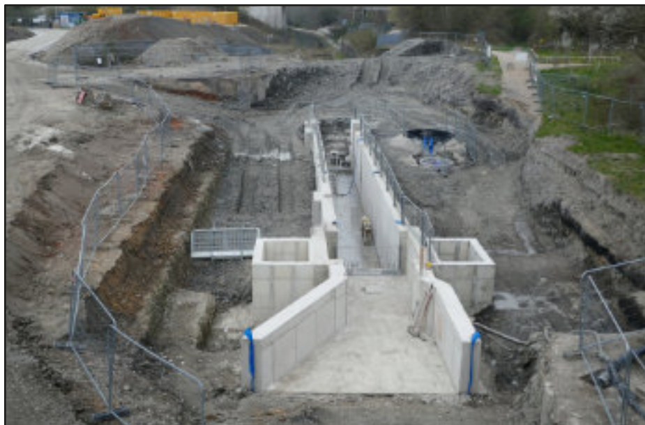
Concreting is complete on the new Keith Ayling Lock chamber; lower wing walls and paddle chambers
