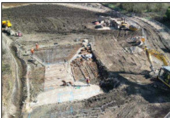
Foundations being laid for the new Bellhouse Bridge
