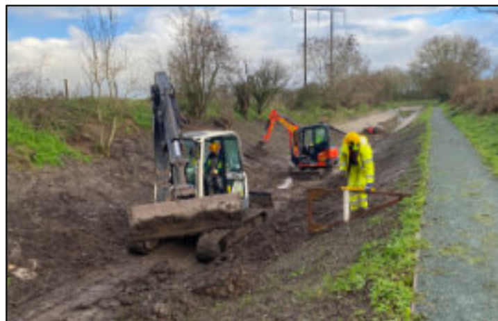
Channel profiling under way on the relatively dry Phase 2 section
