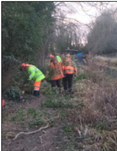
Cutting up and clearing felled vegetation
