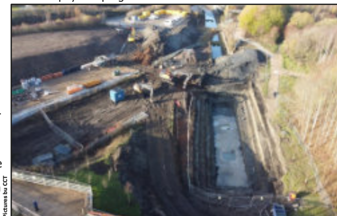
Excavation under way for the new Keith Ayling Lock
