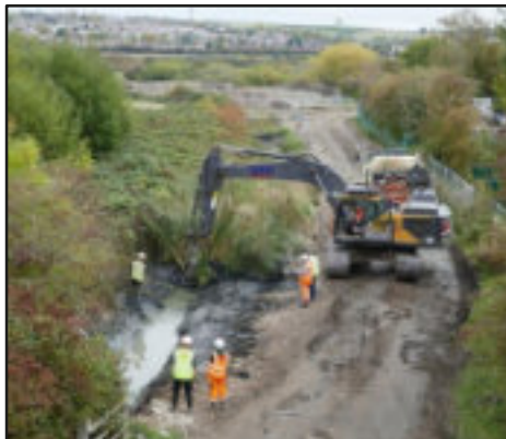
Clearing the channel towards Bellhouse Lane
