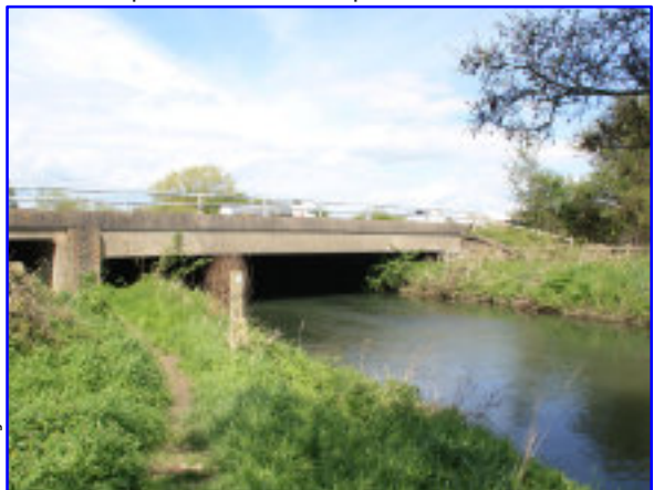
The new length of canal bypassing the Missing Mile will share this existing bridge under the M5 with the River Frome
