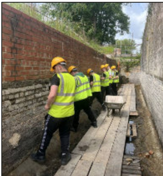
Our Wilts & Berks project: Pewsham Bottom Lock
