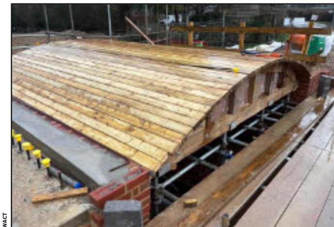
Arch formwork in place at Rooks Hill Bridge, site of 2025's camps
