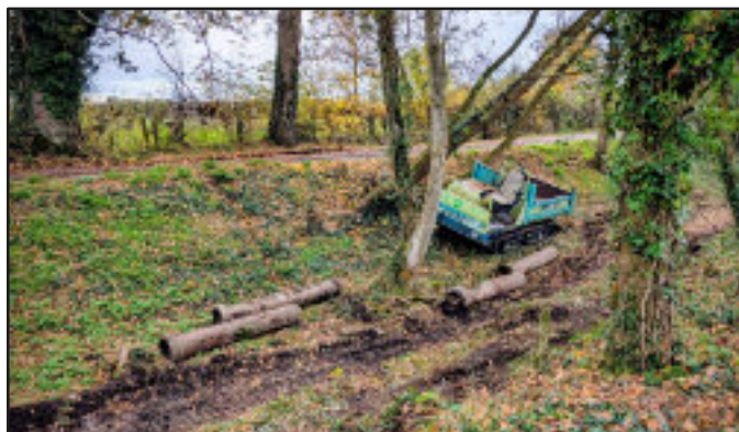
Removing the pipeline laid in the canal bed after it closed
