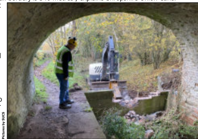
Headwall removal under Malthouse Bridge
