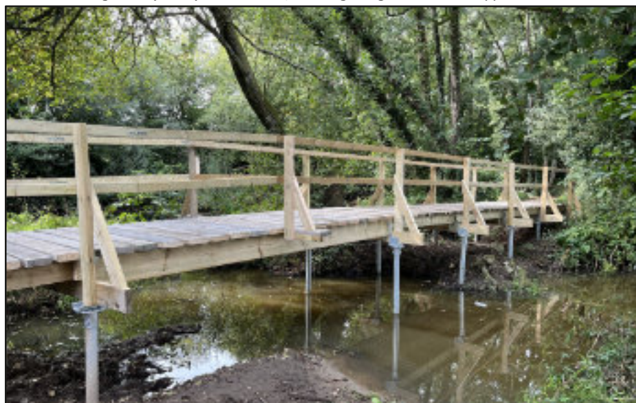
The old bridge and (below) the new one, showing the ground screw supports underneath it
