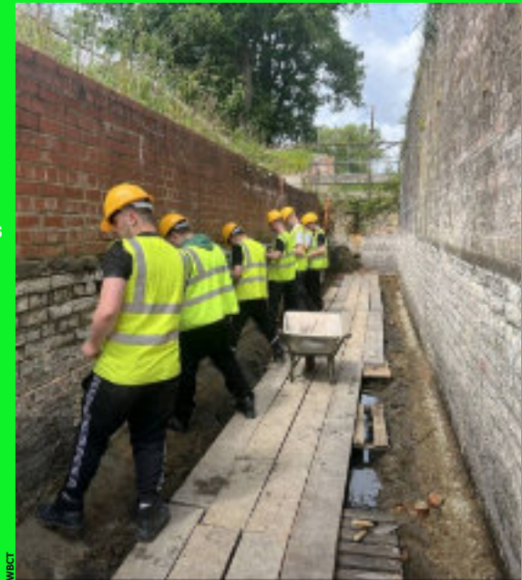
Pewsham Bottom Lock's brickwork receiving attention
