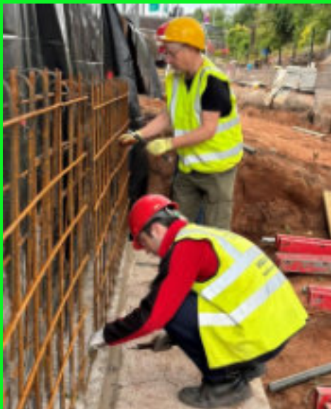
Channel construction near Gallows Wharf
