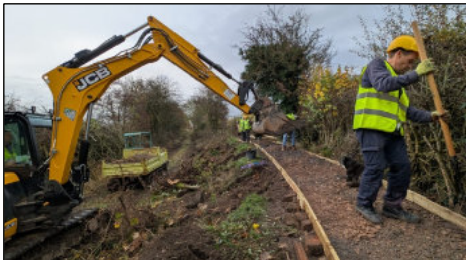
Constructing the towpath
