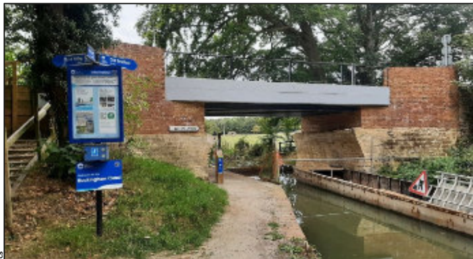
The Buckingham Canal's approach: steel beams and concrete deck on remains of old abutments
