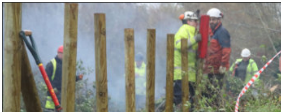
The Site B fence-post bonking crew in action alongside Grove Bottom Lock
