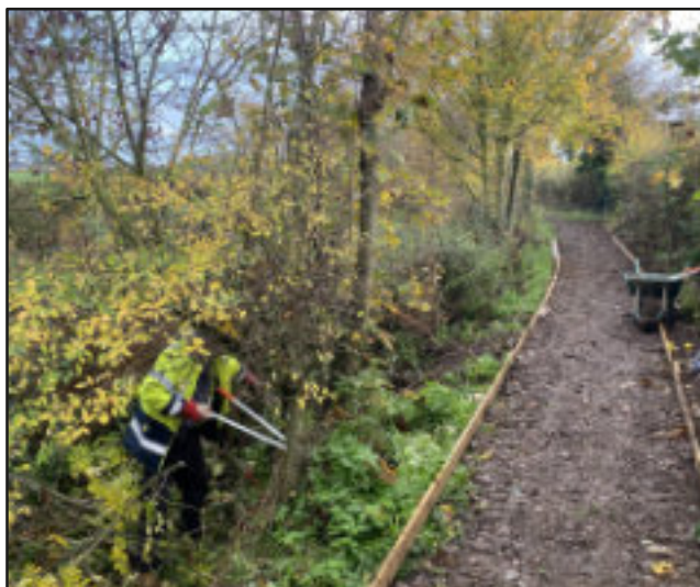
Removal of vegetation in the channel prior to surfacing the towpath
