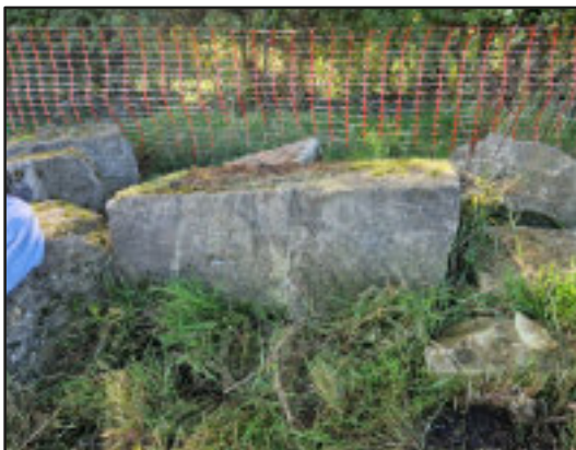
These huge coping stones now need cutting down and placing on top of the walls to finish the work off
