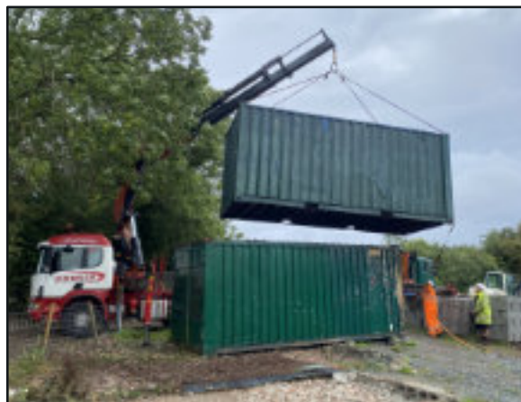
The site compound containers depart for their new home
