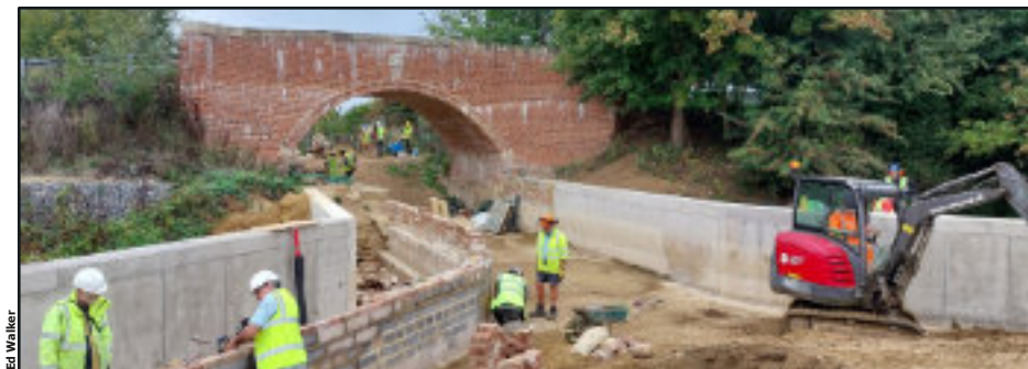
Traditional rebuilt bridge meets modern concrete channel at Weymoor on a London WRG / Kescrg dig
