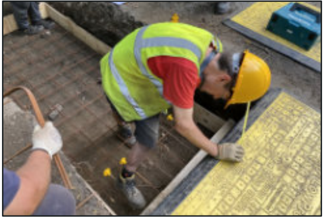
The culvert: preparing to cast a section of the concrete base...
