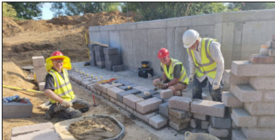
With the completed concrete wall visible behind, construction of the blockwork towpath wall begins
