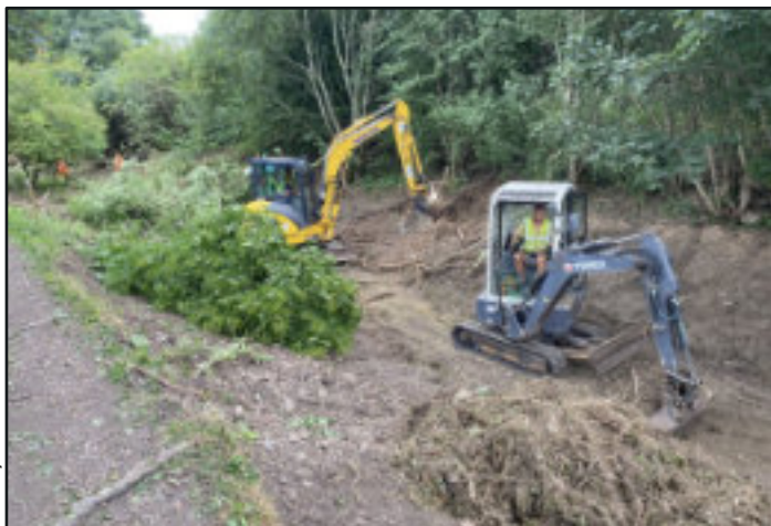
Removing small trees from the banks of the Phase 2 section in August
