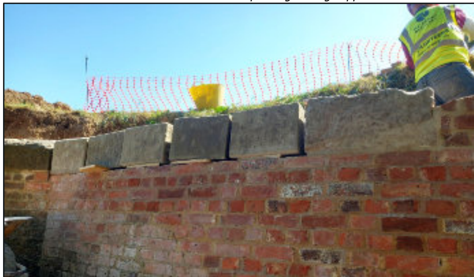
Expertly cast new coping 'stone', and (below) the old and new stones in place, but with the new ones not mortared in pending heritage approval
