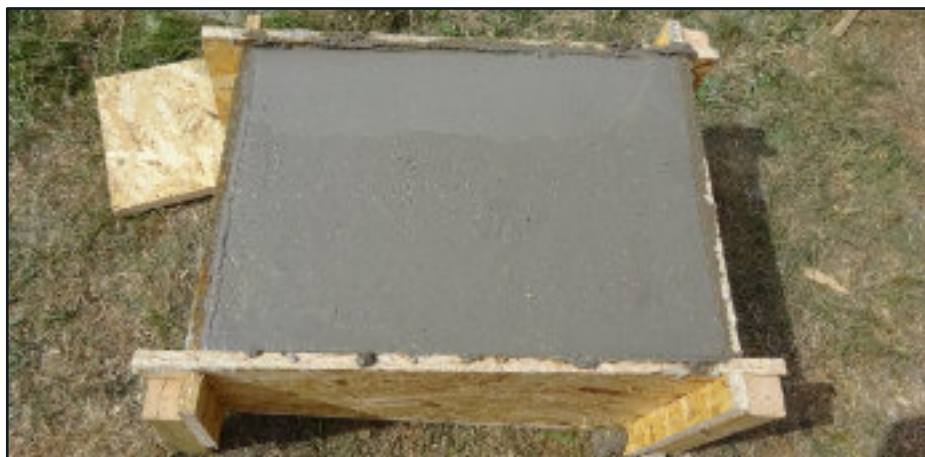
Expertly cast new coping 'stone', and (below) the old and new stones in place, but with the new ones not mortared in pending heritage approval
