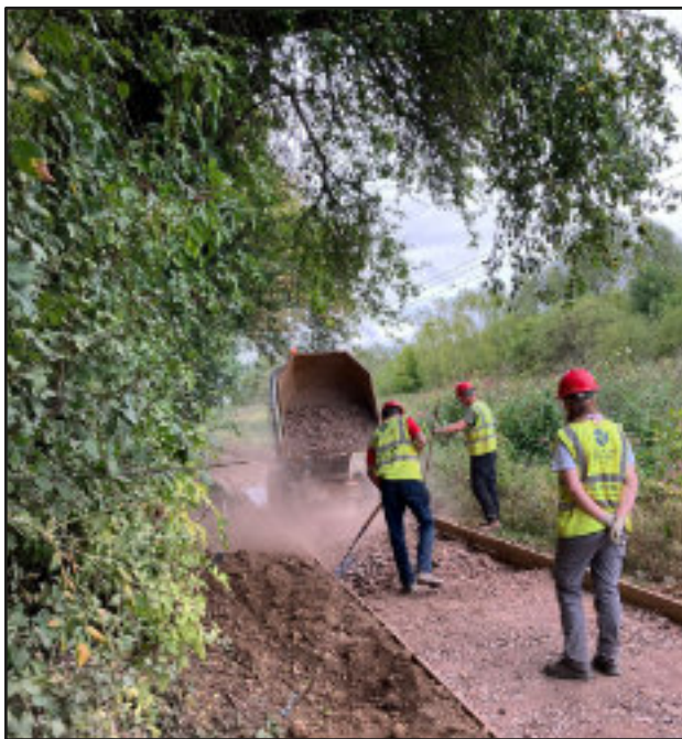
The other job: towpath surfacing by the Cotswold Outdoors Centre
