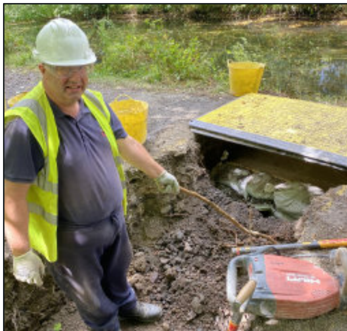
Excavation under way for the culvert under the towpath
