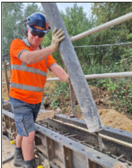
The concrete is pumped in
