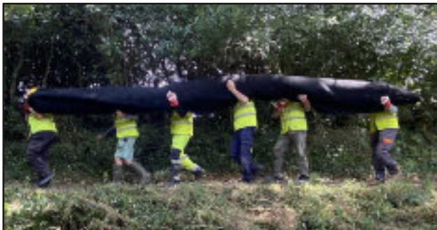
'Carpet caterpillar' transporting the lining material to the work site
