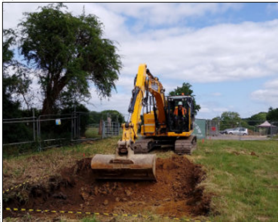
Start of excavation on the Rooks Hill bridge site on 16 June...
