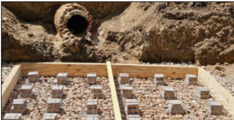
Ready to pour the concrete base for the culvert extension and exit chamber
