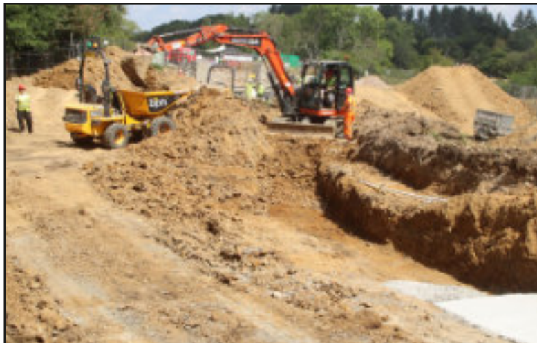
Excavating the foundation trench for the canal wall - note concreted section (right)
