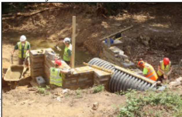
...and the structure nearing completion on the final day
