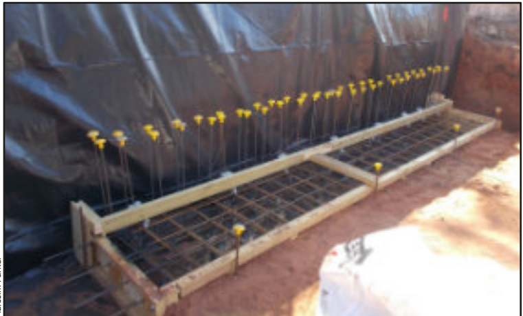
The reinforcement and shuttering are set up ready for the base concrete pour
