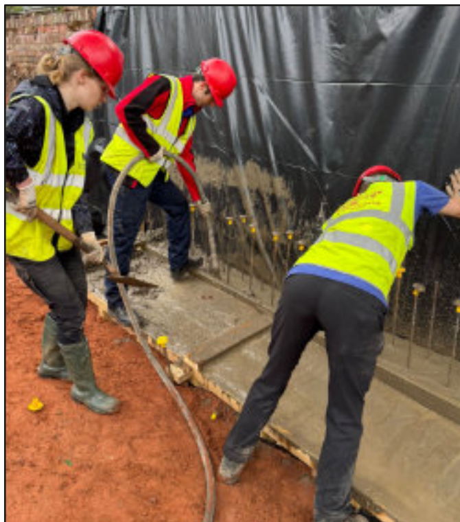
The concrete is poured and vibrated into place
