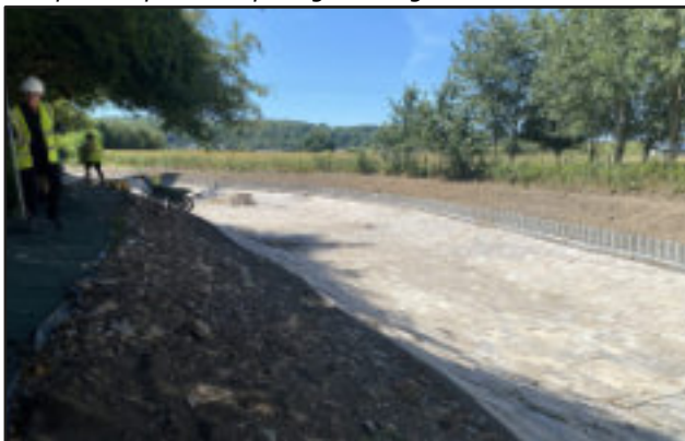
The finished channel
