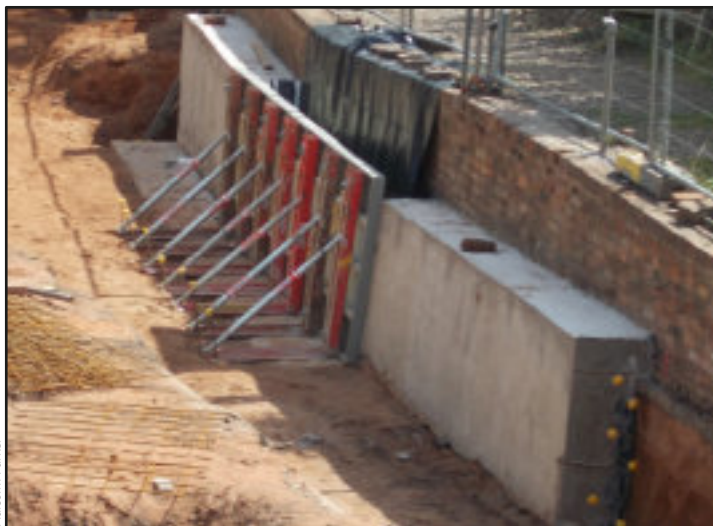
Shuttering for the wall is set up on top of the base
