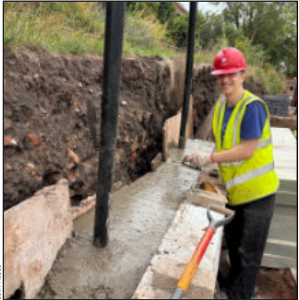
The concrete for the wall is poured and levelled
