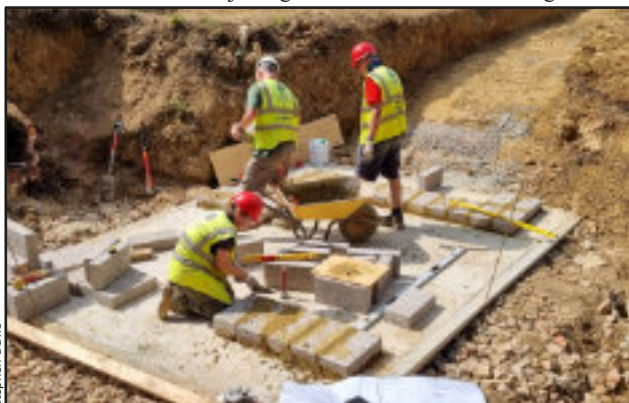
Starting work on the culvert outfall chamber...
