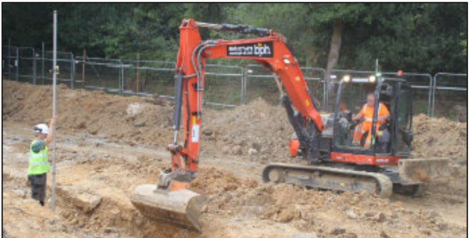
Checking the depth of excavation for the foundation trench
