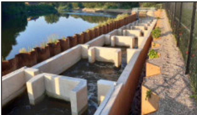
Installing fish passages: one of the 'Unlock the Severn' fish-passes
