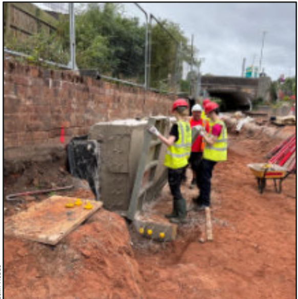
Shuttering is removed to reveal the completed wall section
