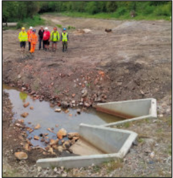
The team, the flood water storage pond behind them, and headwalls of culverts installed in 2023 in the foreground
