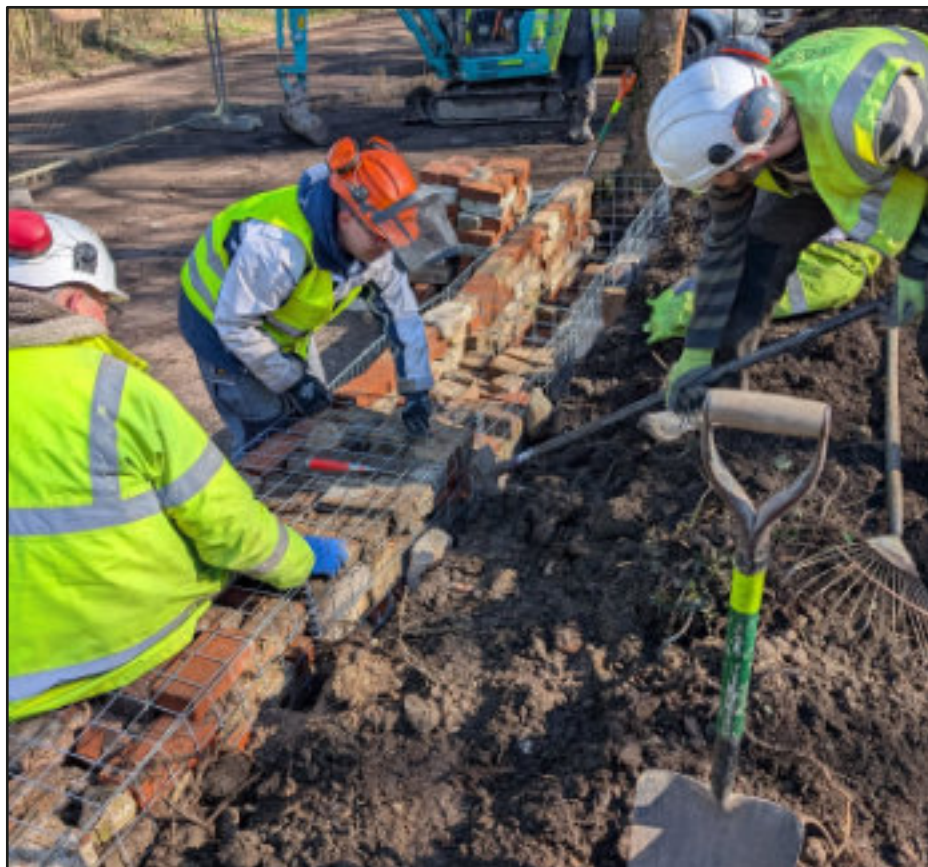
Making up gabions for bank support at Pike Lock on the Cotswold Canals in March
