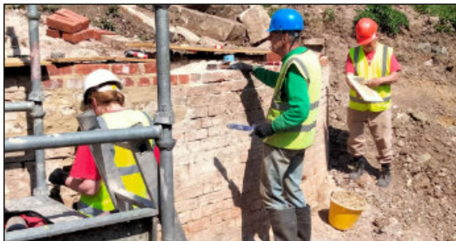
Rebuilding and repointing work on the lock's upper wing wall
