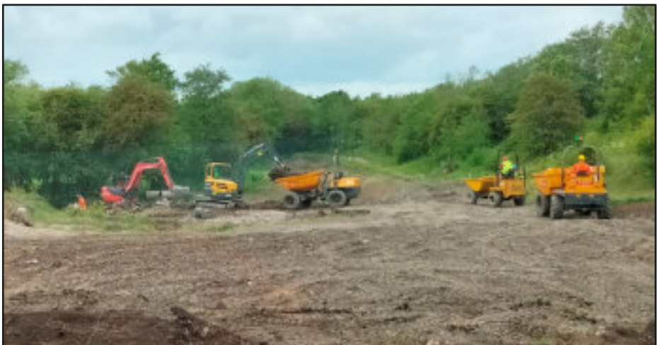
Just some of the machinery: there was also a third excavator and a sheep's foot roller (see back cover)
