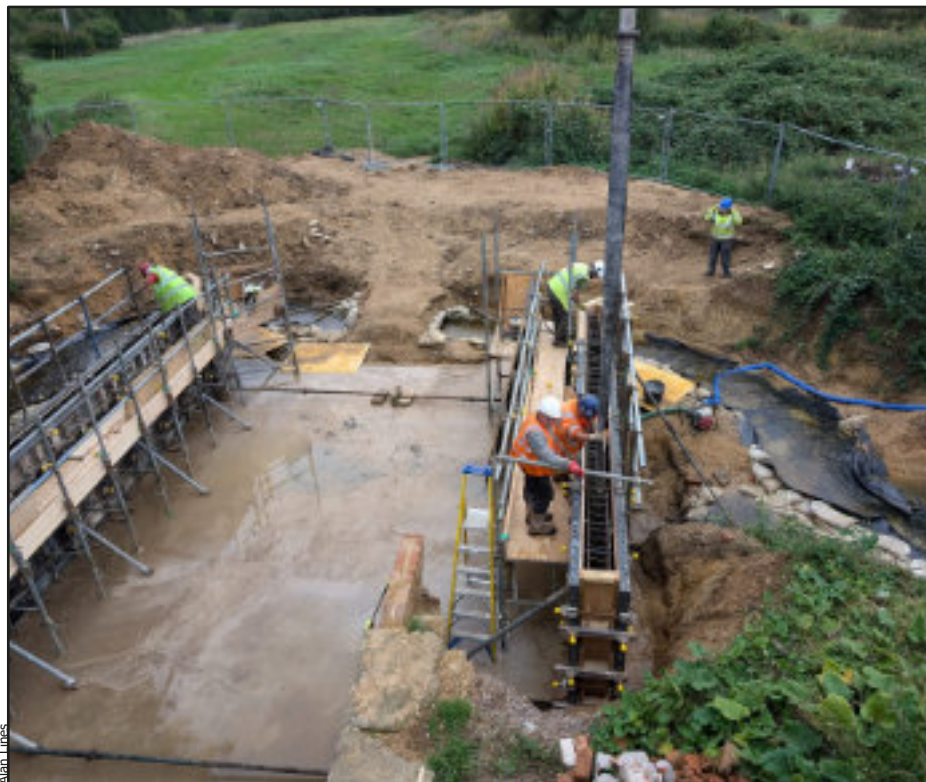
The concrete pour goes in on the final day at Weymoor on the Cotswold Canals in September
