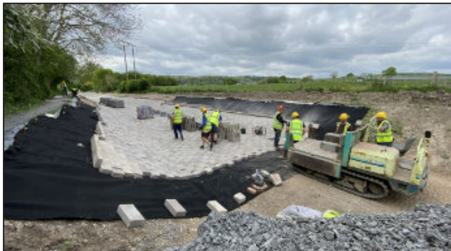
The channel widens considerably on a bend, enough for some soft banking to be installed
