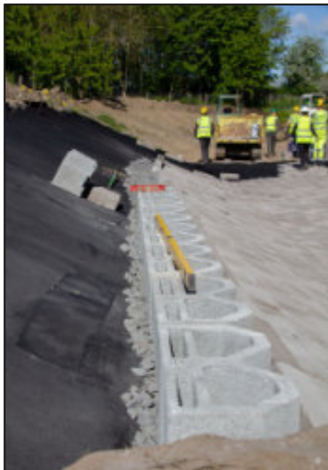
First of two courses of blocks on the soft bank
