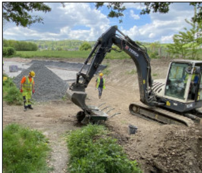
Covering the riprap with soil
