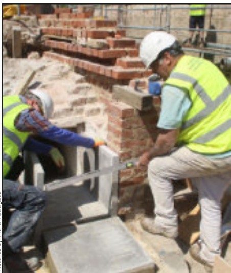
Constructing a top ground paddle culvert
