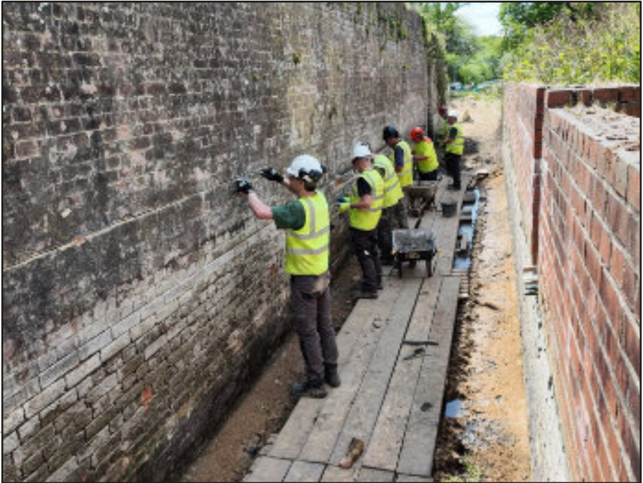
Back to an old favourite: chamber repairs at Pewsham Locks on the Wilts & Berks in May
