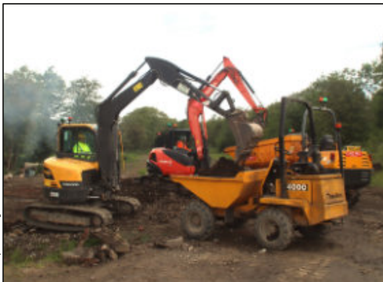
Muck-shift in progress
