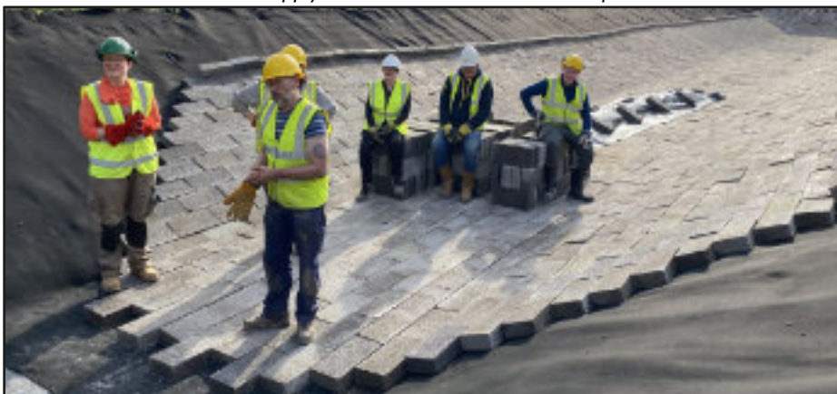
Progress with lining and blocking by Sunday afternoon of the March working party
