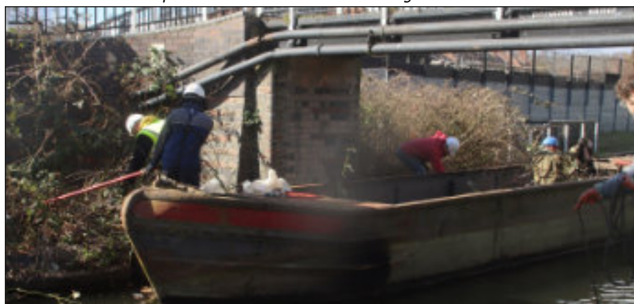
New job for this year: clearing overhanging vegetation on the offside of the canal
