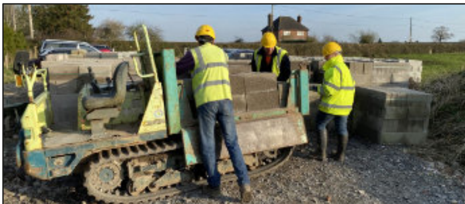
A constant supply of blocks loaded from the compound
