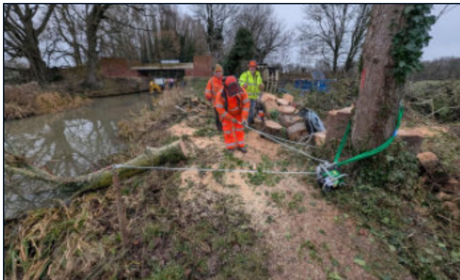
Using WRG Forestry's new powered winch to drag felled trees out of the canal by the rebuilt Bridge 1
