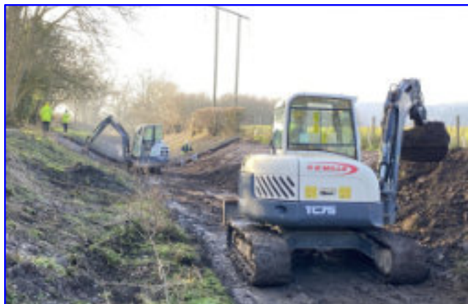
Profiling the lined section of channel
