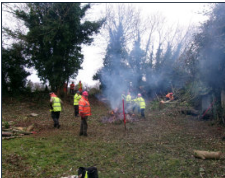
Clearing the 'triangle', the site for the disabled access visitor car park
