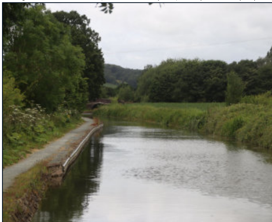
The Montgomery Canal, restored with a hard towpath bank, but a vegetation fringe on the opposite side
