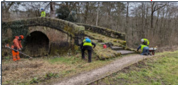
Volunteers clearing the restored Bridge 70
