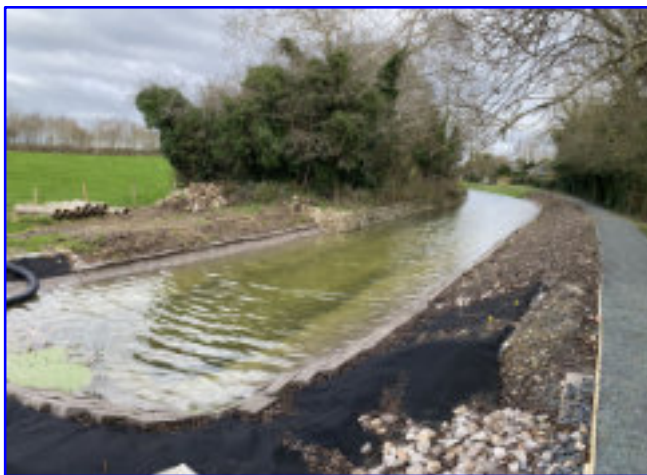
Completed channel section filling up after December's rain
