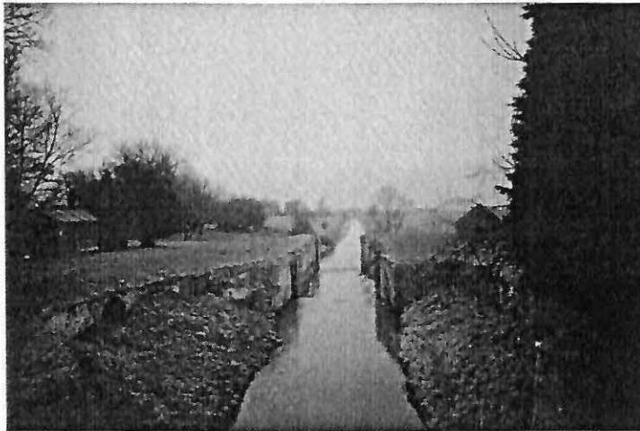
Barrel sided lock at Alvingham Lock on the Louth Navigation
