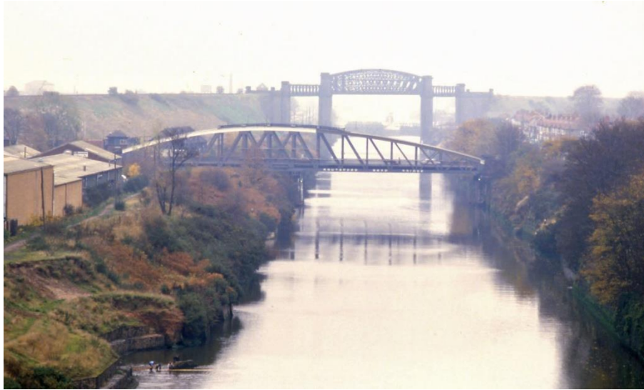
Knutsford Road Swing Bridge and beyond Latchford Railway Bridge seen from the Cantilever Bridge in 1984.
