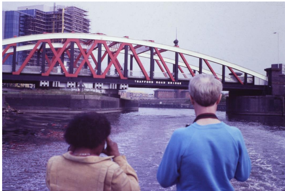
Trafford Road Swing Bridge in 1992 before it was fixed in position, looking towards the bend to Pomona Docks.
