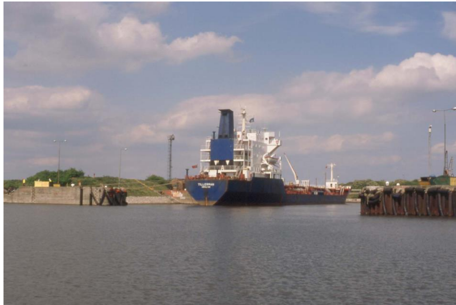
Stanlow Oil Dock seen from the east 1998
