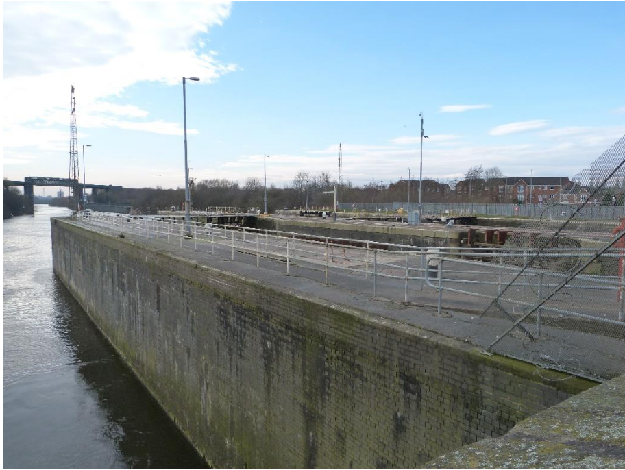
Irlam Locks seen from above the lock weir and looking west 2016.
