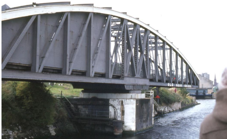
Old Quay Swing Bridge 1983.
