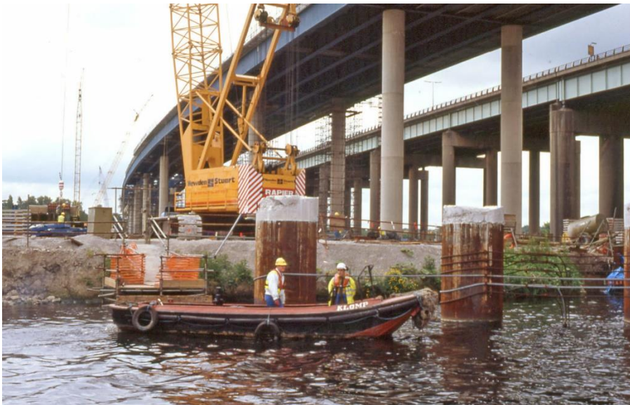
Second Thelwall High Level (M6) crossing under construction in 1994.
