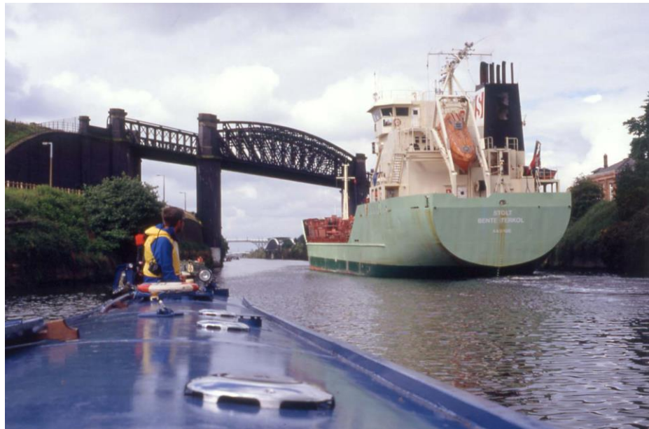
Latchford Railway Viaduct taken from a boat about to enter Latchford Locks. Knutsford Road Swing Bridge and the Cantilever Bridge can be seen beyond 1994.
