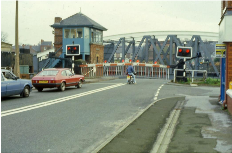
Chester Road Swing Bridge seen from the Warrington side 1984.
