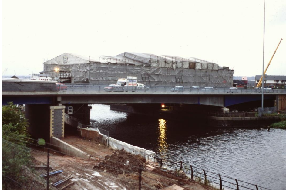
Trafford Road Fixed Bridge, with the swing bridge encapsulated behind 1997.
