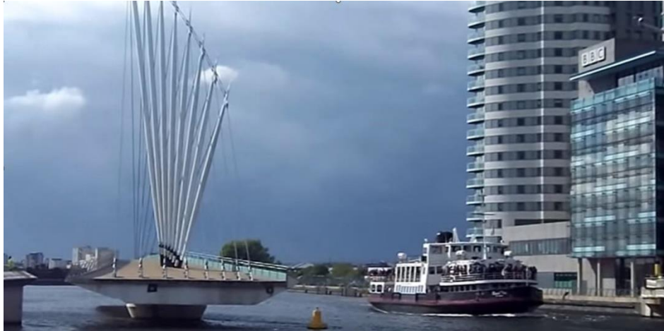
Media City swing footbridge swung to allow a Mersey Ferry to leave Mode Wheel Locks and pass "Media City".
