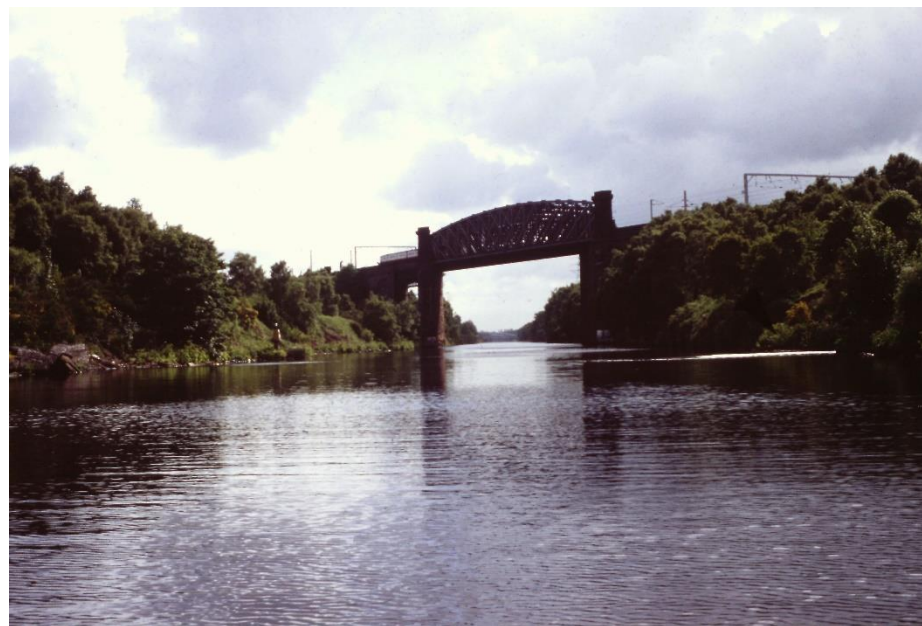
Acton Grange viaduct in 1994.
