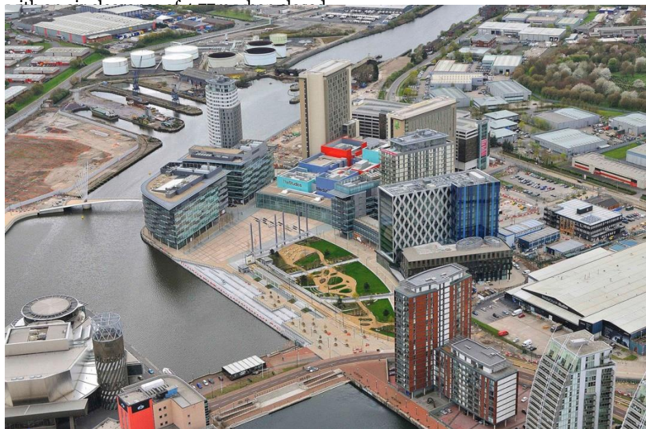
From Peel Ports Web Site – Media City, Manchester Dry Docks, Media City Swing Bridge, and the stub of what used to be Salford Dock 9.
