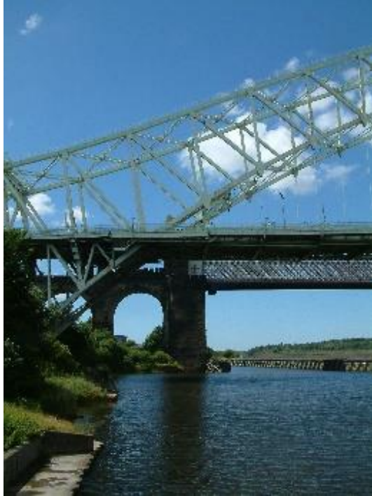
From the east, the end of the Silver Jubilee Bridge and the Railway Viaduct over the Manchester Ship Canal 2004 seen from the footings of the former Transporter Bridge.
