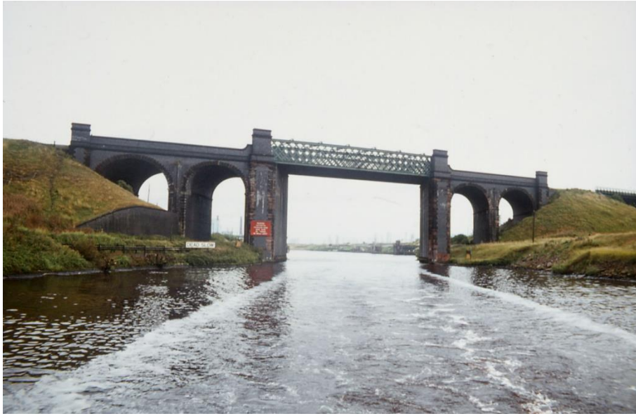
Cadishead Viaduct from the west 1977.
