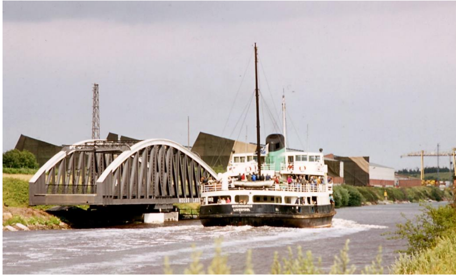
Manchester-bound Mersey Ferry "Overchurch" at Moore Lane 1978.
