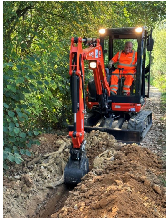
Adrian S in digger number 1. Photo: Tim Lewis
