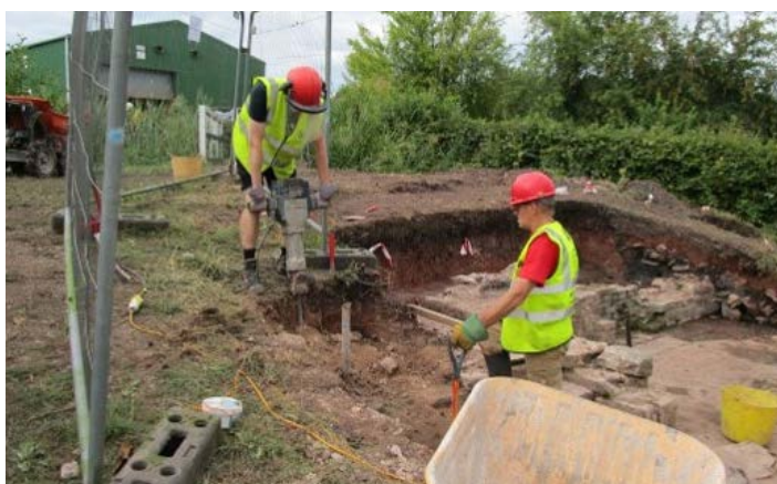
Breaking out a concrete base to a scaffold tube.
