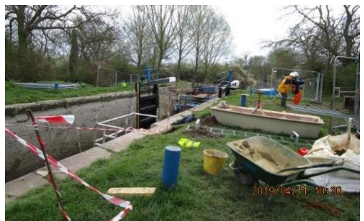
Work to a dewatered lock chamber without edge protection.
