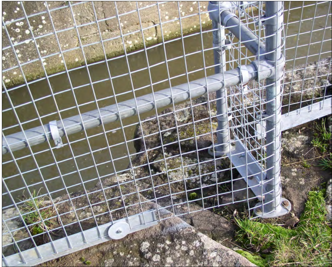
Photograph 10.5: Example of the Quoins at Thornton Lock
