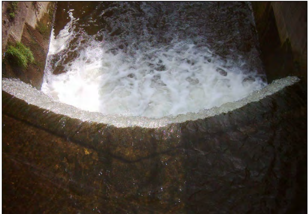
Photograph 10.4: Top Sill of Roughton Lock
