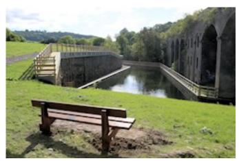
excavated and the waste material placed behind the piling. A concrete channel separates the River Frome from the new line of canal.
