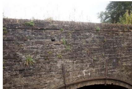
Area of generally reasonable pointing with isolated local loss
