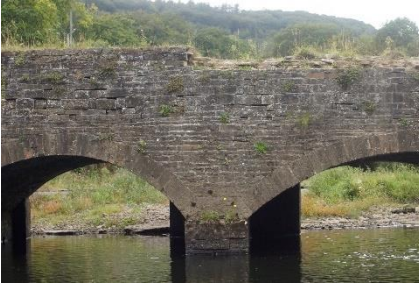
Sparse soft vegetation growth from outside face of downstream channel wall (D).
