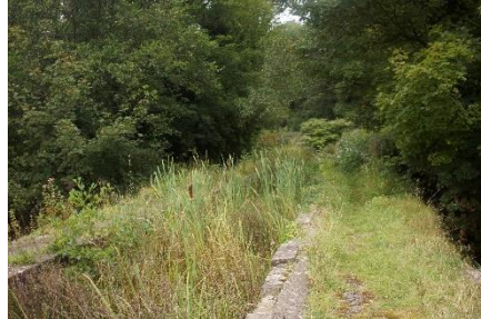
Dense soft vegetation growth in canal channel (E) and variable growth on downstream channel wall head (D and H).
