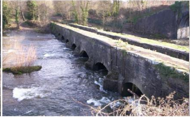
Aberdulais Aqueduct, North side
