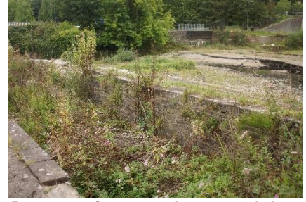
Dense soft vegetation growth in canal channel (E) and moderate growth on inside face of upstream channel wall (C).
