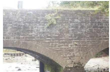
Area of generally reasonable pointing
