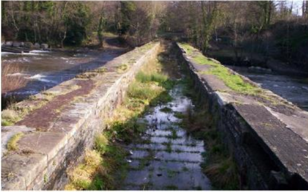
Aberdulais Aqueduct looking East
