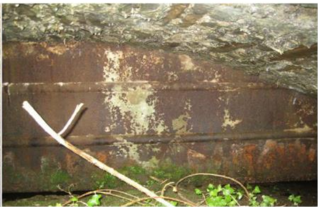
Aberdulais Aqueduct, iron trough
