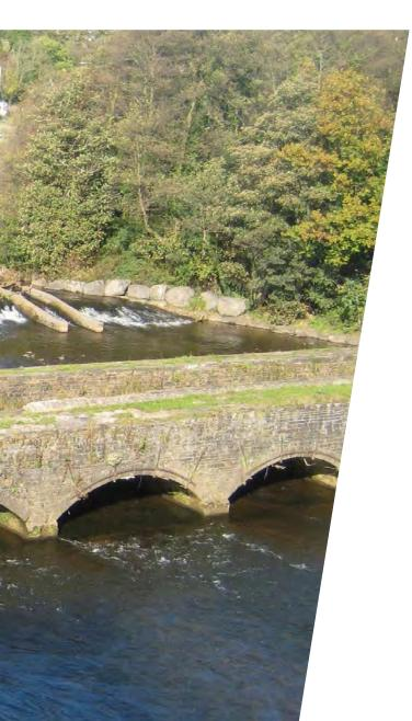
In early 2020, Storm Dennis caused further damage to the aqueduct and the low arches were overwhelmed by floodwaters. Debris built up and some masonry was swept away.
