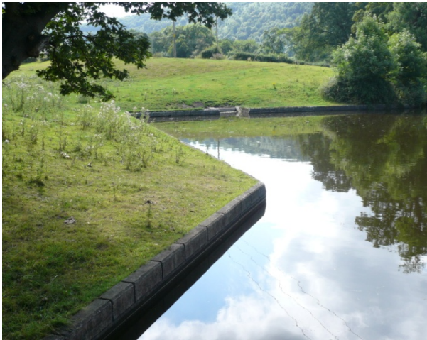
Unfriendly winding hole – concrete, sharp corners (Llangollen Canal)
