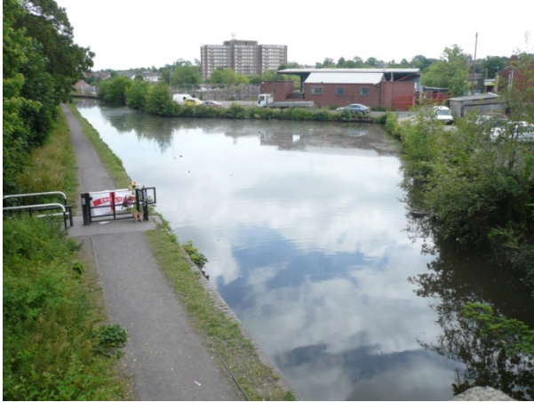
Winding hole with generously wide vee angle (Langley Green, BCN)
