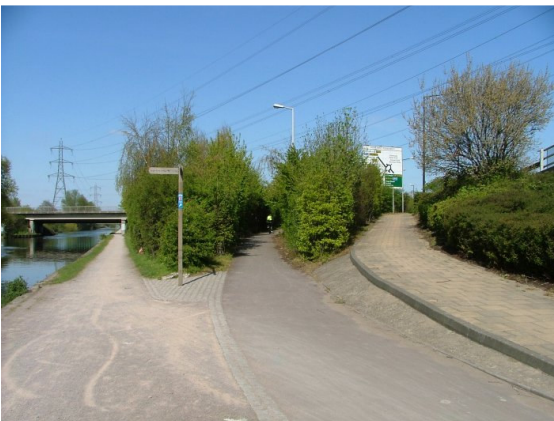
Separate access for cyclists and pedestrians at Edmonton
