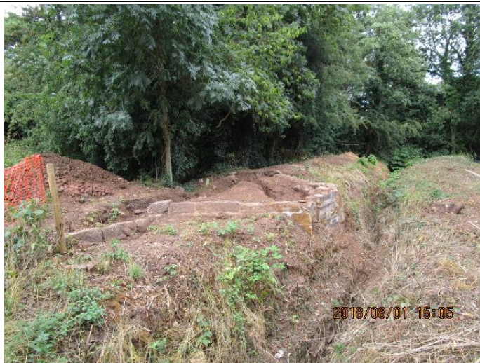
Photo of weir after 2018 canal camp
