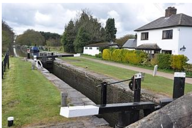
Shade House Lock, Trent & Mersey Canal.
