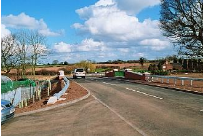
Cappers Lane canal bridge on completion in 2006
